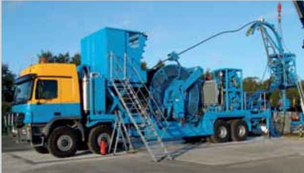
Truck Mounted CTU Operation
